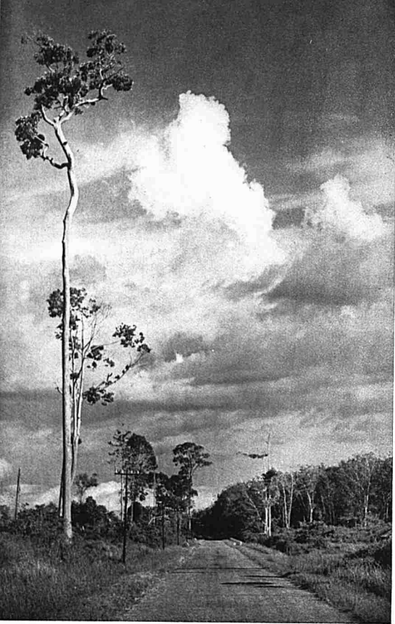
The Dindings Road between Bruas and Sitiawan
